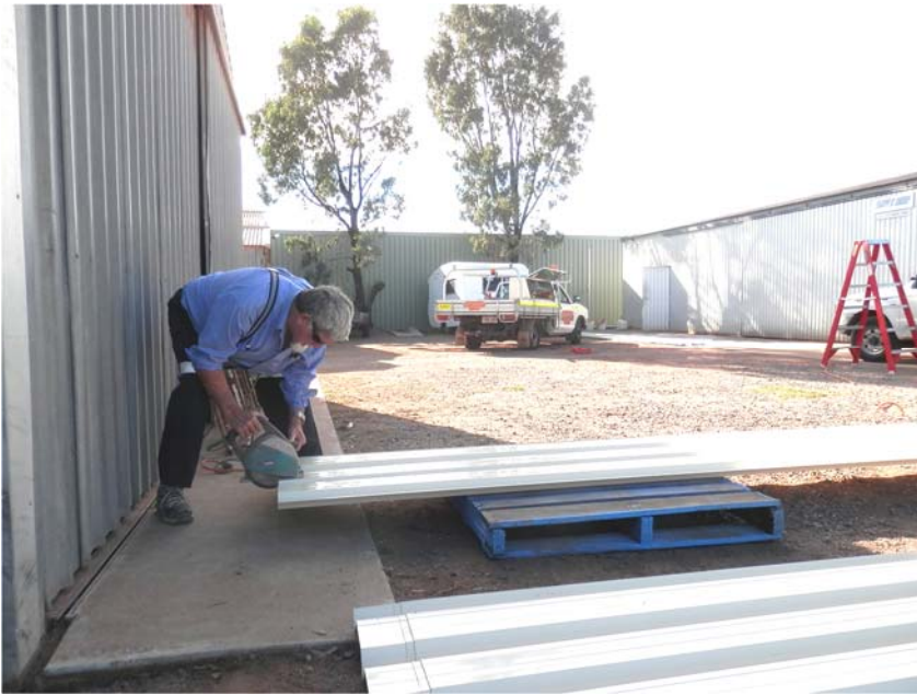
Peter Strawbridge trimming the colorbond roofing sheet
