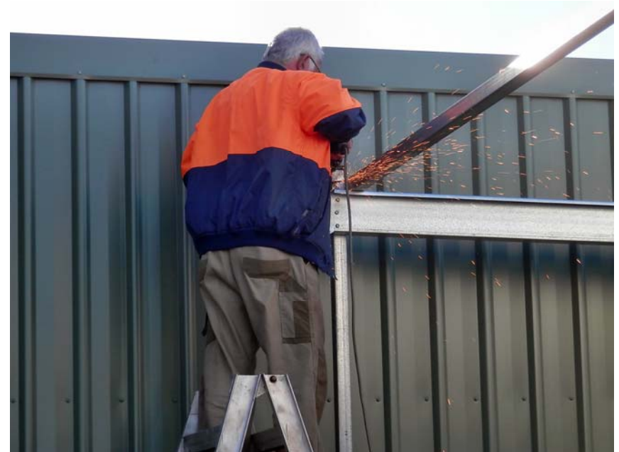
Ron cutting (trimming) the support poles
