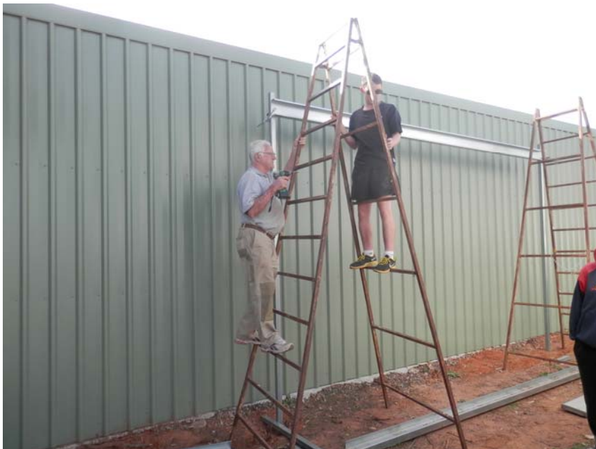
Ron Snr and Jnr just secured the first 'C' Column
