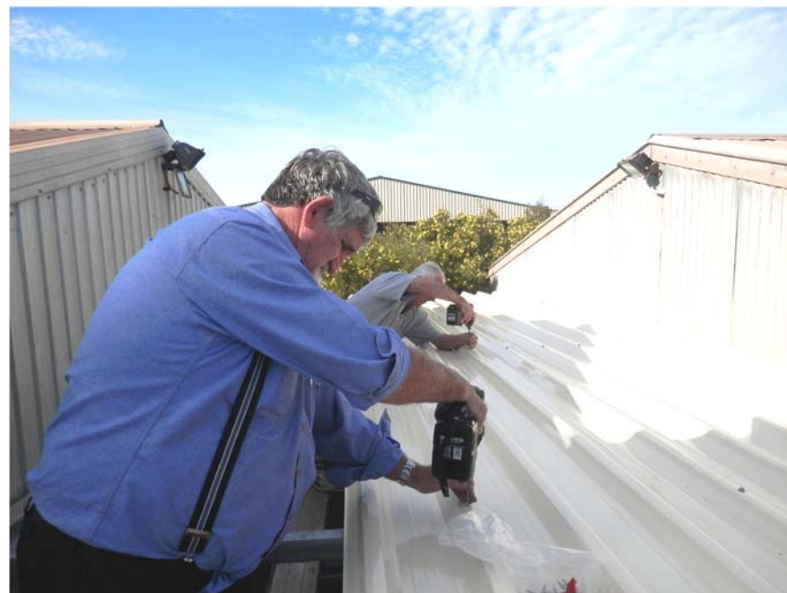
Peter Strawbridge and Ron King fastening down the roof
