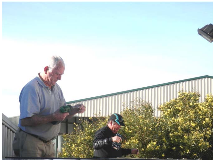
Ron King and Andrew Strawbridge fastening down the roof
