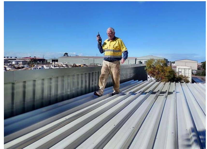
Securing the colorbond roofing sheets
